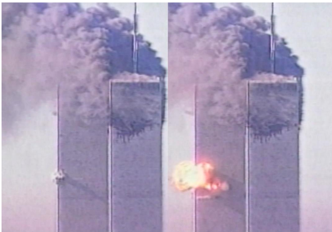
Figure 2: Flight 175 exit point with developing fireball very close to the NE corner of the building. Note also the higher and well-centered entry scar in the North Tower.
