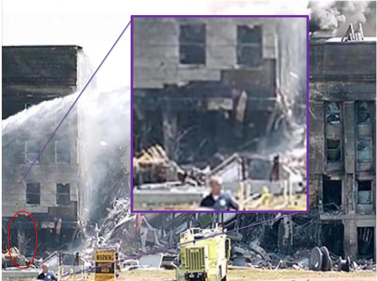
Fig. 11 – Column 9AA is irreversibly shown to be bowed directly east
