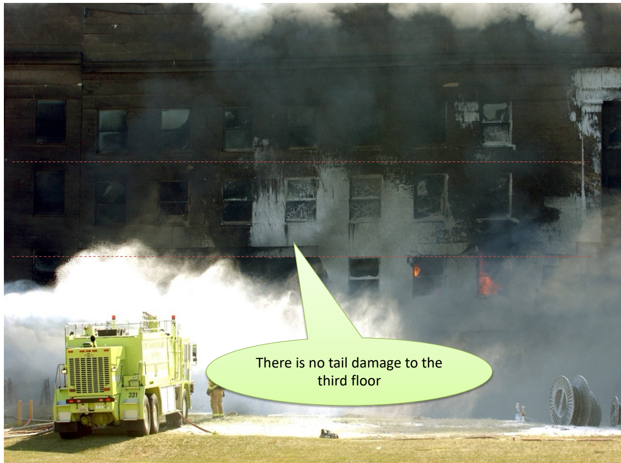
Fig. 4 – USMC Cpl. Ingersoll captured intact 3 rd and 4 th floors at the 14 th column line
