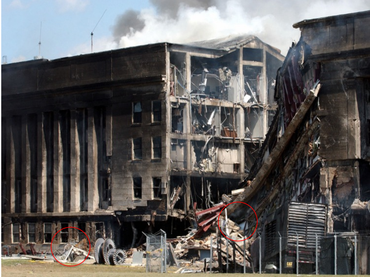
Fig. 23 – Image of event aftermath, with broken retaining wall on left and dislodged generator on right
