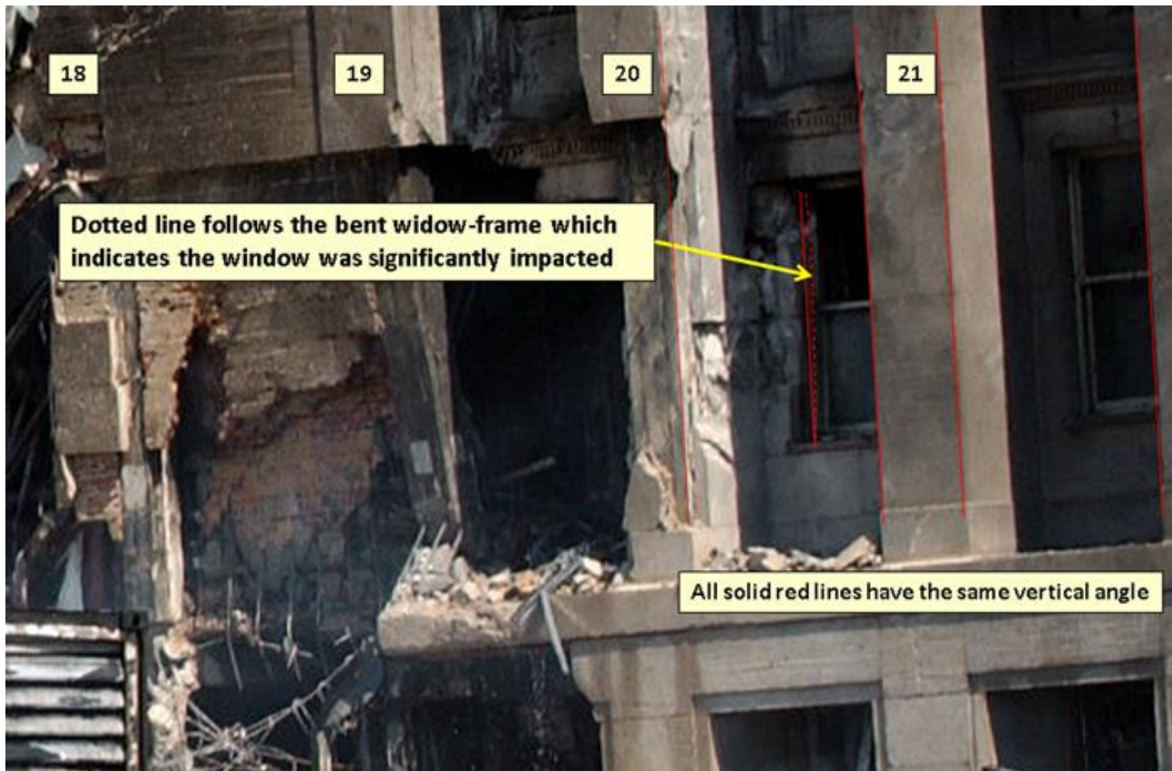
Figure WC15: Wayne Coste figure 15, damage between C20 and C21
