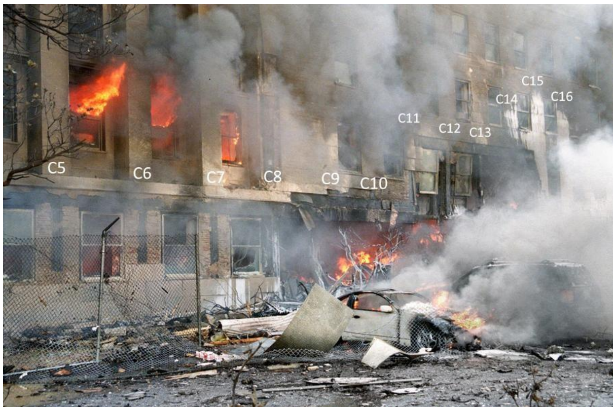
Figure 9: Explosion overpressure damaged Windows in the outer ring E between columns 5 and 8.
