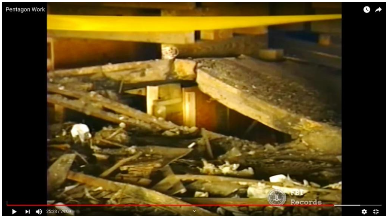
Figure WC26: Wayne Coste figure 26, Uplifted floor slab
