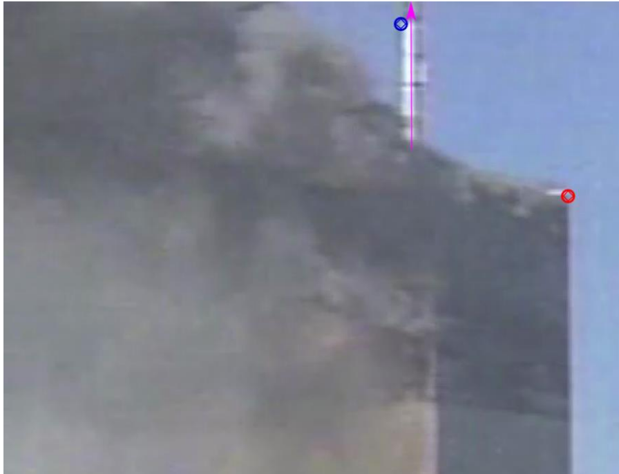
Figure 11 The blue and red markers are used for tracking the relative motion of the antenna and roofline. The magenta arrow is a vector placed along the lower section of the antenna to measure the apparent tilt angle of the antenna.
