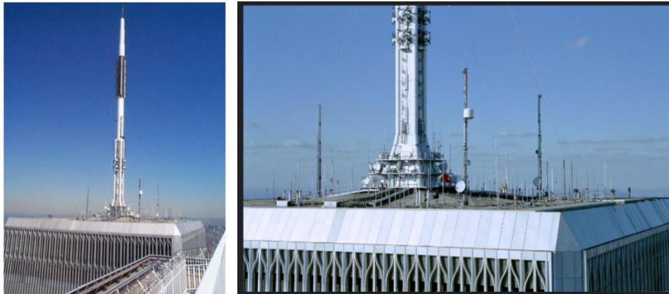
Figure 7 The antenna on the North Tower highlighting its connection to the roof structure.
