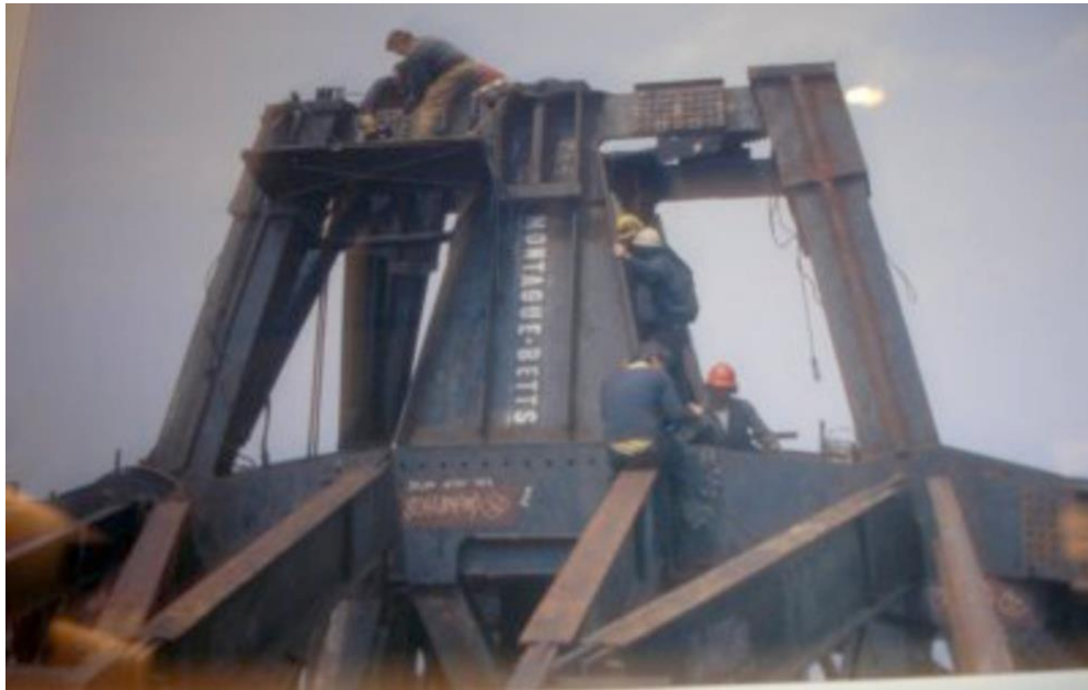
Figure 4 Base of the antenna attached to the hat truss system.
