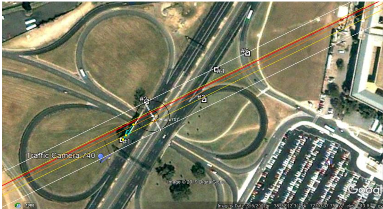
Figure 3 Precise location of the flight path through the light poles with the right engine (yellow line) impacting the front quarter of the generator trailer.
