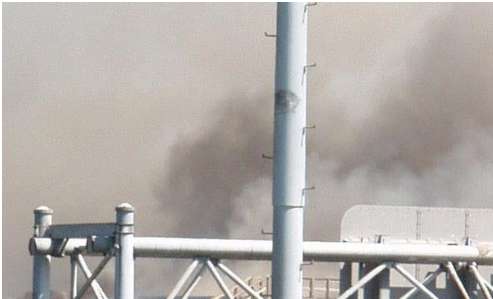
Figure 10 Detailed view of scar and missing rung on freeway traffic camera zoomed and cropped from Staff Sgt Gary Coppage Photo.
