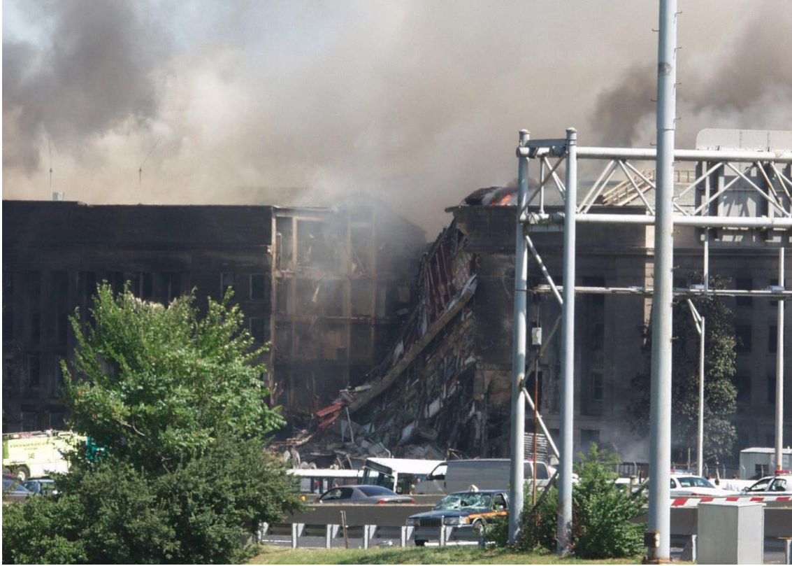
Figure 9 A photograph taken by Staff Sgt Gary Coppage shows a notch cut out of the tree on the left and a scar and missing run on the VDOT traffic camera pole at the top right. Note that this photograph was taken at least a half hour after the impact because the roof of the Pentagon can be seen to have collapsed.
