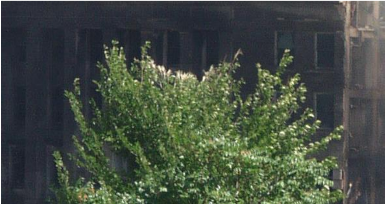
Figure 2 Detail view of tree notch, showing the frayed ends of the stems.
