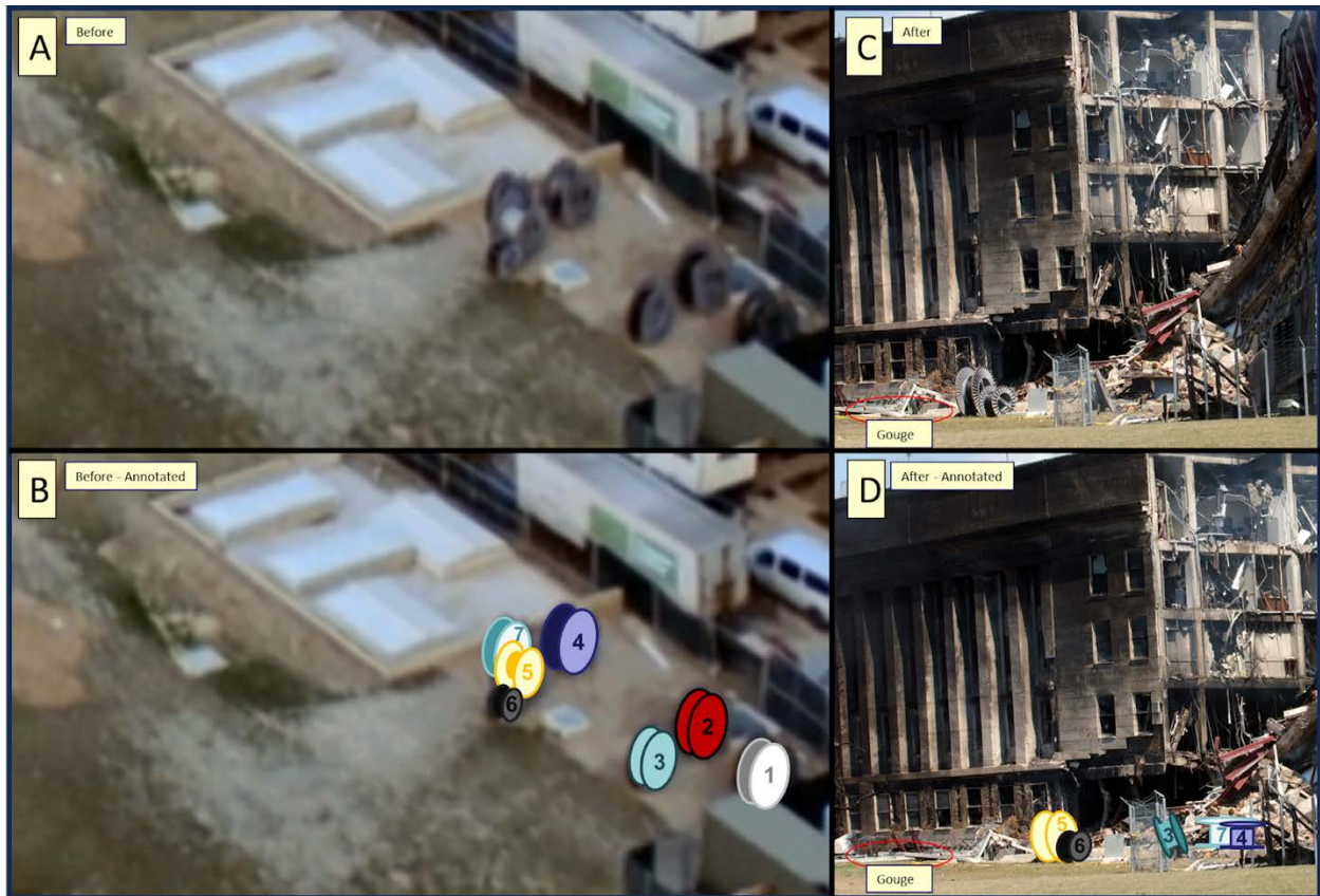
Figure 12: Location of wire spools before and after impact.
