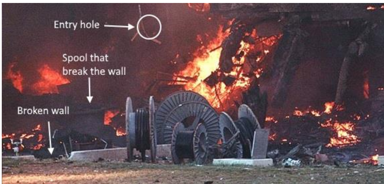
Figure 10: Broken ventilation wall and the cable spool that crossed it.
