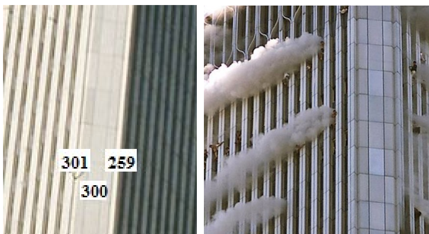
Figure 4: On the left, the northeast corner of the South Tower with columns labeled. Photographed by Gulnara Samoilova. On the right, a close-up of one of the chamfered corners of the North Tower. Photographed by Jose Jimenez.
