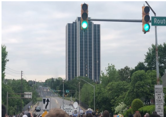
Figure 1: The Martin Tower moments before it was demolished by explosives.
