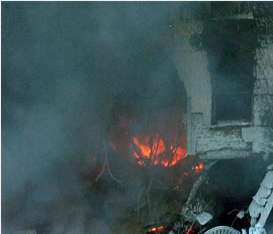
Figure 11: Fire is visible where Column 14 should have been attached to the second-floor slab, proving the slab was missing and the column was detached.
