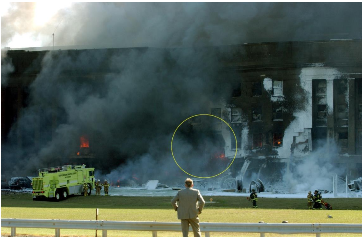
Figure 8: Jason Ingersol photo showing the extensive damage to the first floor. The "small opening" of the cropped image is hidden behind smoke, above and slightly to the right of the spectator's head. For reference, the large slanted column on the first floor is Column 16.
