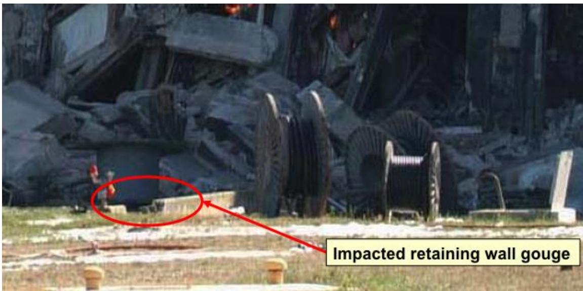
Figure 18: The notch in the retaining wall locates where the left engine nearly touched the ground. The wing was sufficiently high to pass over the cable spools.
