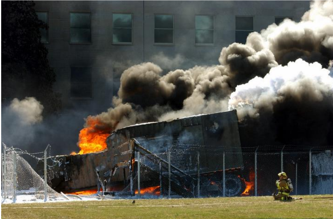
Figure 20: The fence is damaged in the path of the right engine but not elsewhere.
