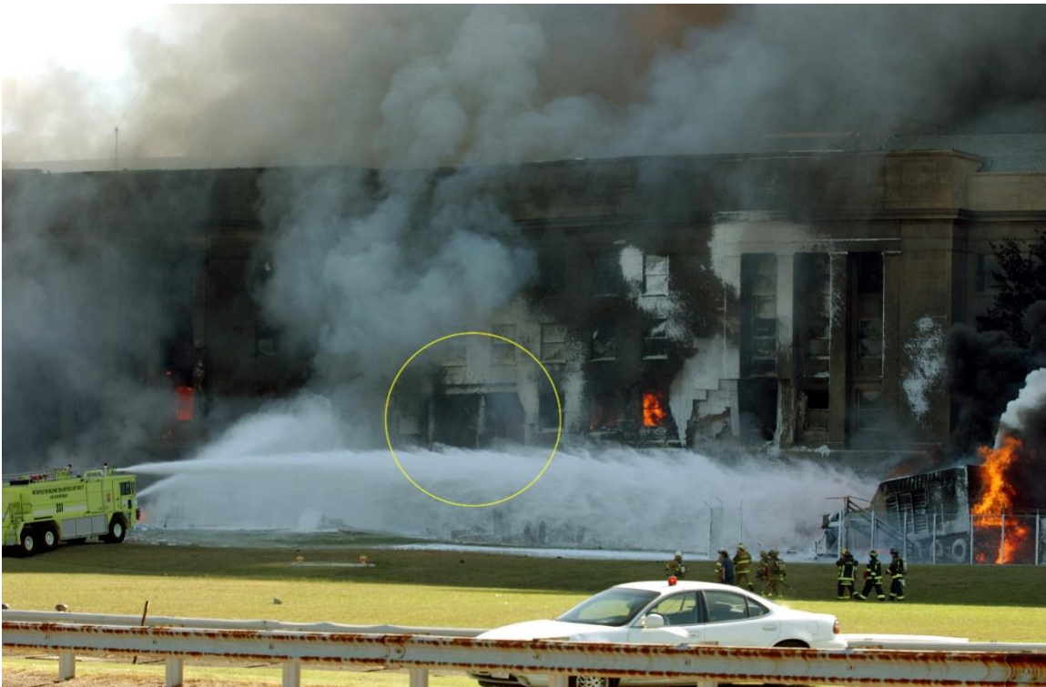
Figure 7: Jason Ingersol photograph from which the small second-floor opening was cropped. The first-floor damage is obscured by fire hose spray.
