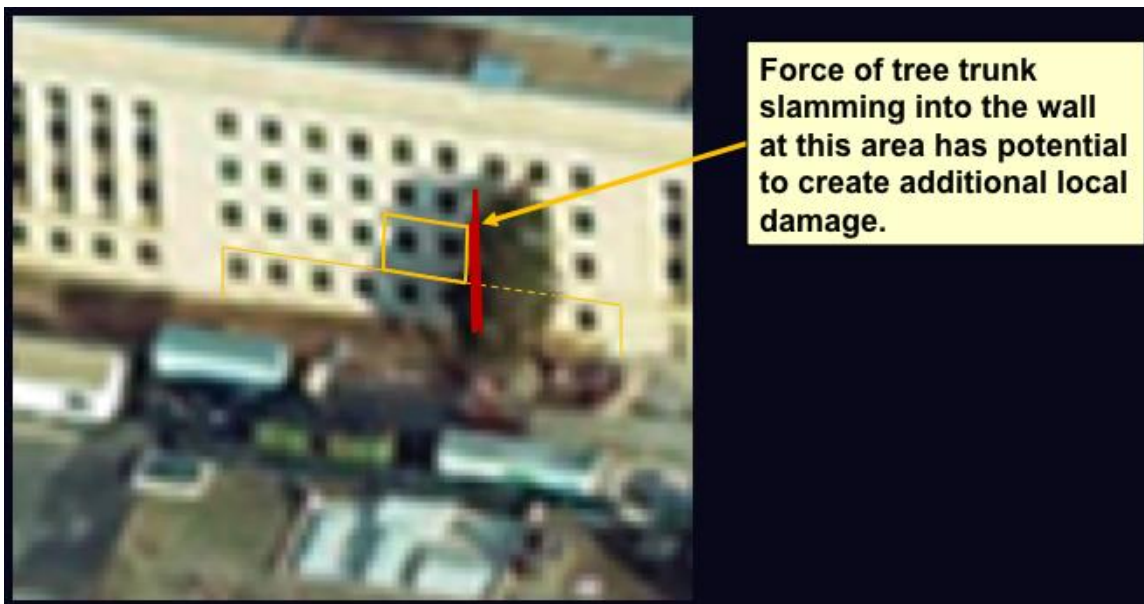
Figure 15: The tree is pushed into the building and northward (leftward) along the wall, which could help account for the elimination of the second-floor wall panels in the vicinity of Column 14.
