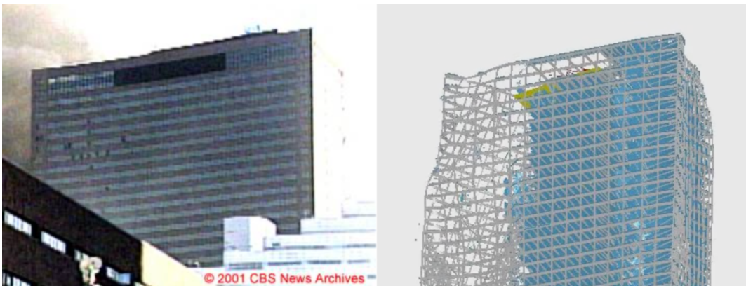
Figure 6: Video and analysis animation at 7.5 seconds after initiation of east penthouse collapse.
