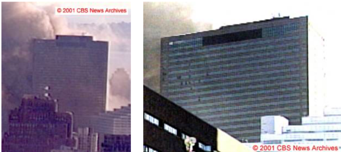
Figure 5–199. Cropped frames from the Camera 2 video clip in Figure 5–185 and the Camera 3 video clip in Figure 5–186, showing the north face of WTC 7 5.0 s ± 0.1 s after the east penthouse began to move downward.
