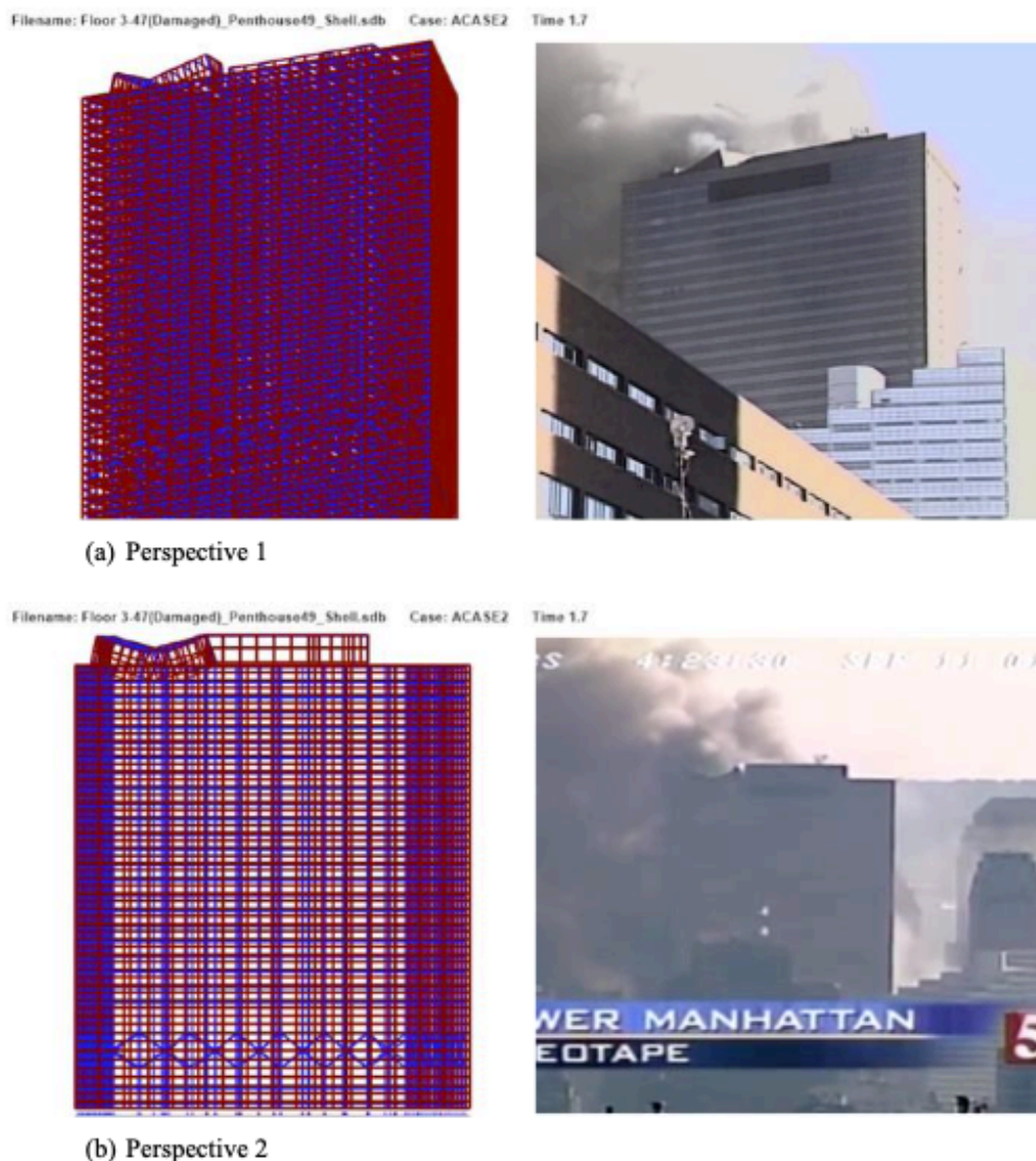
Figure 4.17 (a) Comparison of simulated collapse to perspective 1; (b) comparison of simulated collapse to perspective 2.
