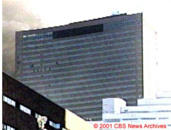
Figure 5–200. Cropped frames from the Camera 2 video clip in Figure 5–185 and the Camera 3 video clip in Figure 5–186, showing the north face of WTC 7 7.5 s ± 0.1 s after the east penthouse began to move downward. The intensities have been adjusted.
