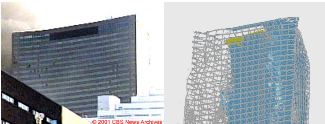
Figure 7: Video and analysis animation at 8.1 seconds after initiation of east penthouse collapse.
