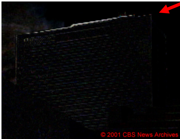
Figure 5–201. Cropped difference frame at 7.5 s ± 0.1 s after the east penthouse began to move, created by subtracting the frame reproduced in Figure 5–199 from the Camera 3 video clip shown in Figure 5–200. The intensity levels were adjusted.
