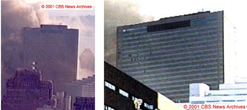
Figure 5–199. Cropped frames from the Camera 2 video clip in Figure 5–185 and the Camera 3 video clip in Figure 5–186, showing the north face of WTC 7 5.0 s \pm 0.1 s after the east penthouse began to move downward. The intensities have been adjusted.
