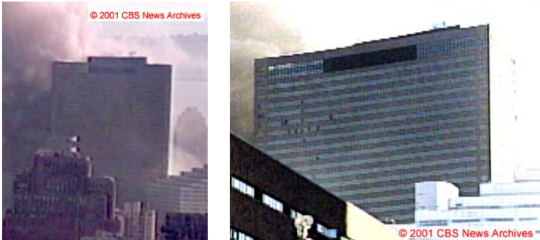
Figure 5–200. Cropped frames from the Camera 2 video clip in Figure 5–185 and the Camera 3 video clip in Figure 5–186, showing the north face of WTC 7 7.5 s \pm 0.1 s after the east penthouse began to move downward. The intensities have been adjusted.
