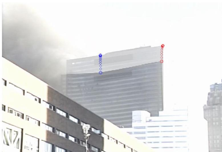
Figure 9: A frame from Camera 3 at 2.3 seconds into the downward motion laid over a frame just before the start of downward motion.
