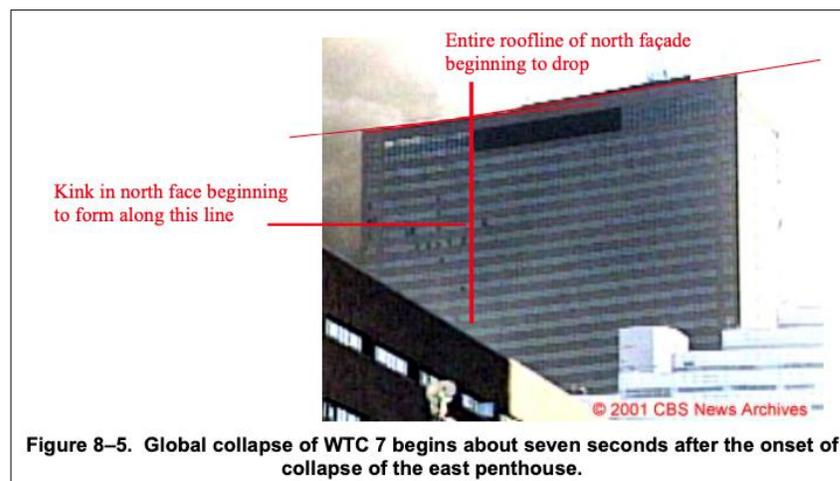
**Thus, the downward motion of WTC 7's north face roofline at the onset of global collapse is more accurately characterized as a sudden transition to free fall.** Prior to the initiation of the entire roofline's free fall, the middle of the roofline dropped approximately half a meter, then stopped, and then dropped approximately 1 meter further, before entering into free fall along with the entire roofline” (Architects & Engineers for 9/11 Truth, 2020, p. 39).
