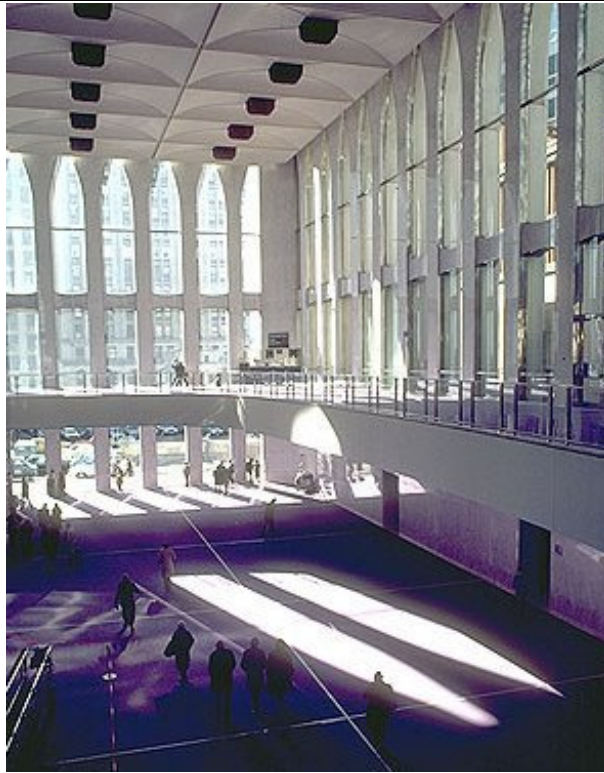
Un-sourced picture of the WTC tower lobby. Notice the location of the cross supports along the exterior column 'tridents' with respect to the ground level.
