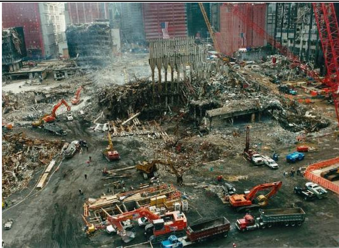
October 17, 2001: South tower. It is evident that debris resided at least in the first few sublevels as well as filling 1 to 2 levels of the lobby based upon this photograph. 45
