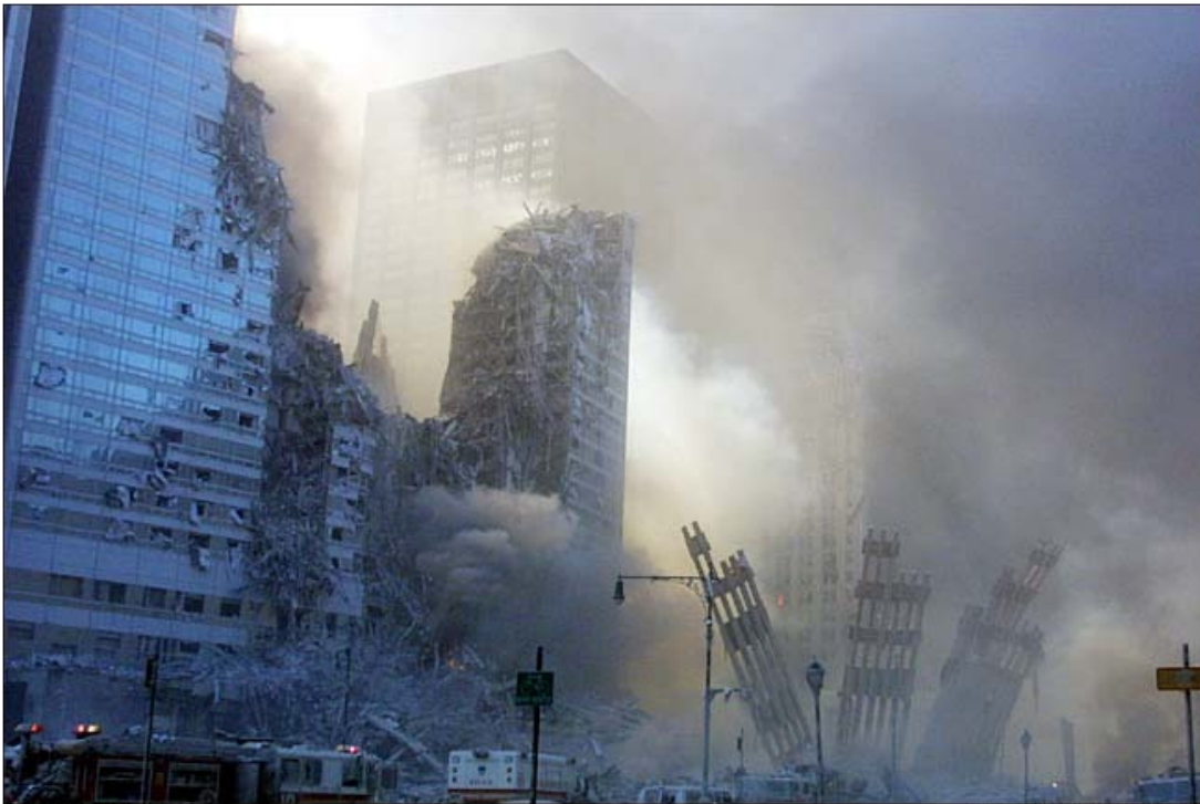
WTC3 after the collapse of the South Tower exhibiting the large vertical slash through it
