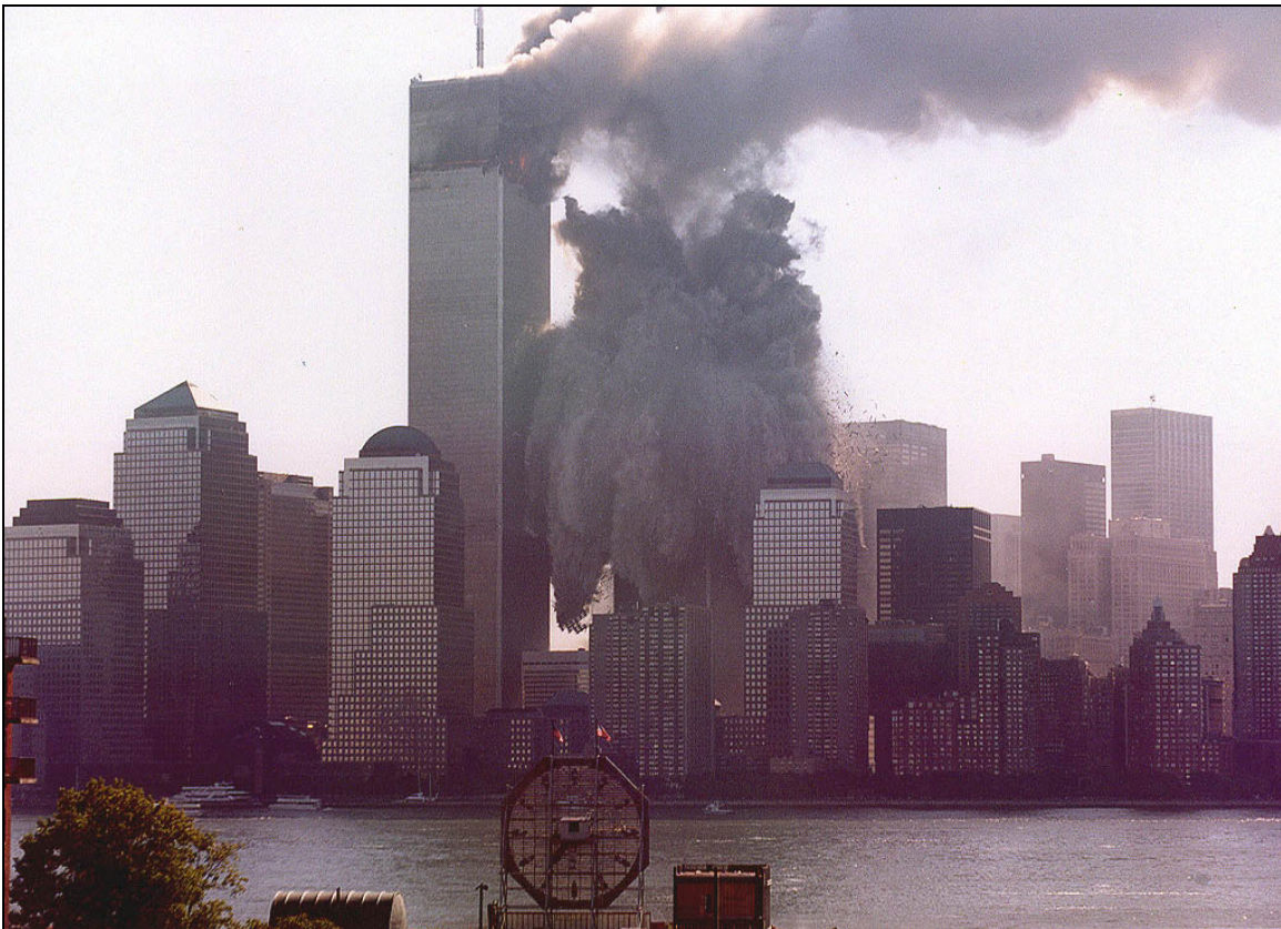
Figure 1: A view from the west of the collapsing south tower.
